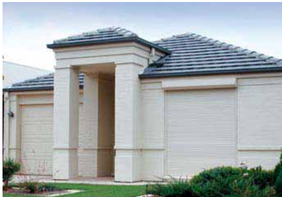
Figure 3.28: Examples of roller shutters over window openings
