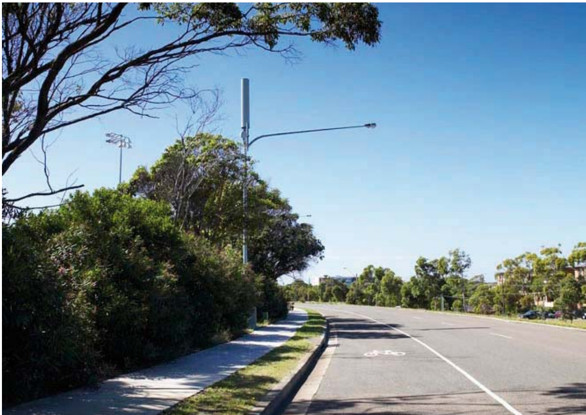
Panel antenna on street light pole
