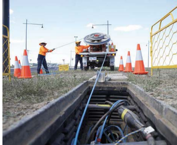
Cable being inserted into duct.
