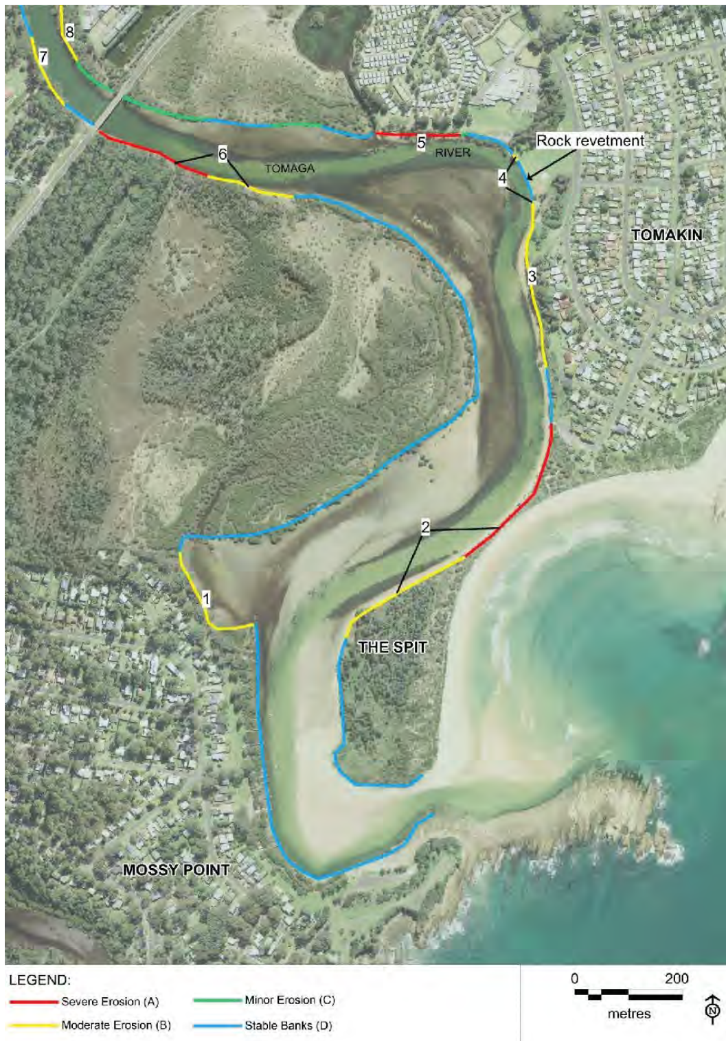
Figure 16: Current areas of erosion lower estuary
