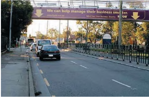
✓ DOES NOT DETRACT FROM ARCHITECTURAL ELEMENTS OF BRIDGE; DOES NOT BLOCK VIEWS; ADVERTISING FORM COMPATIBLE WITH BRIDGE FORM
