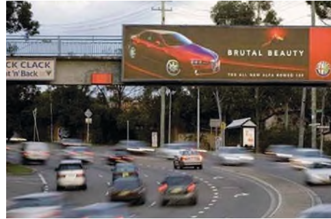
✗ PROTRUDES ABOVE THE TOP OF THE ROAD BRIDGE; NOT IN KEEPING WITH BRIDGE ARCHITECTURE
