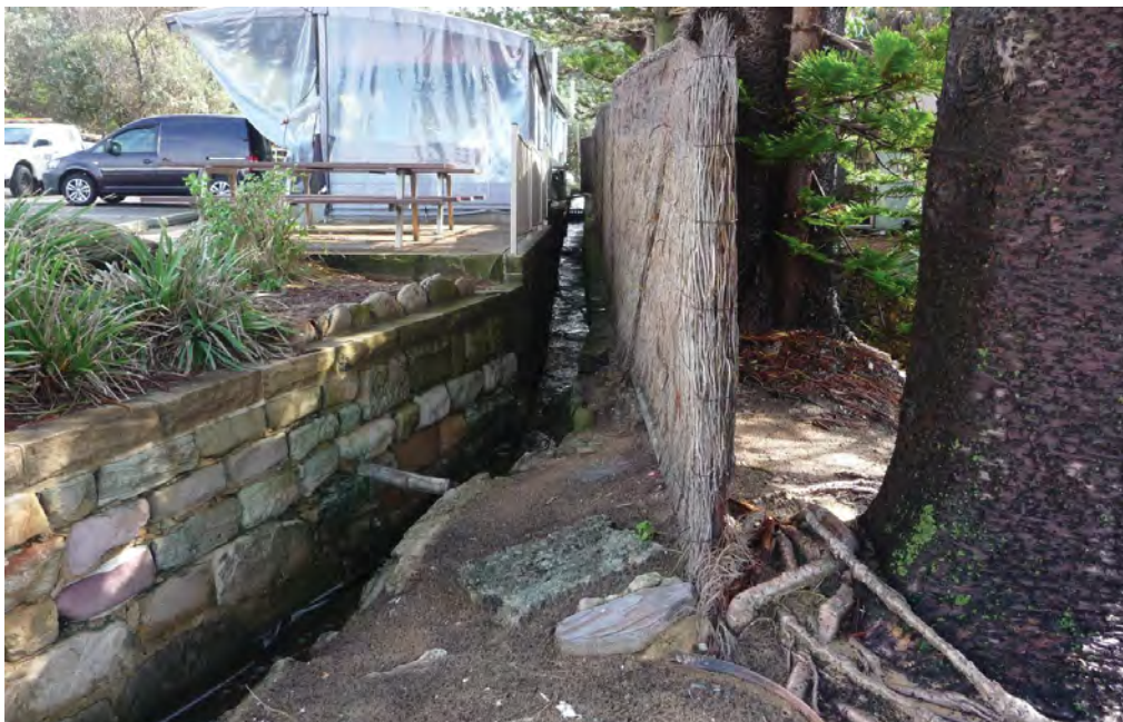
Figure 14: Bilgola Kiosk channel located immediately north of kiosk/café
