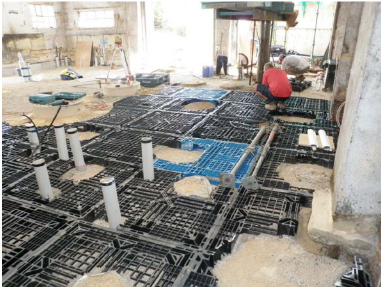
Figure 7 Polypropylene formers create a sub-slab void
