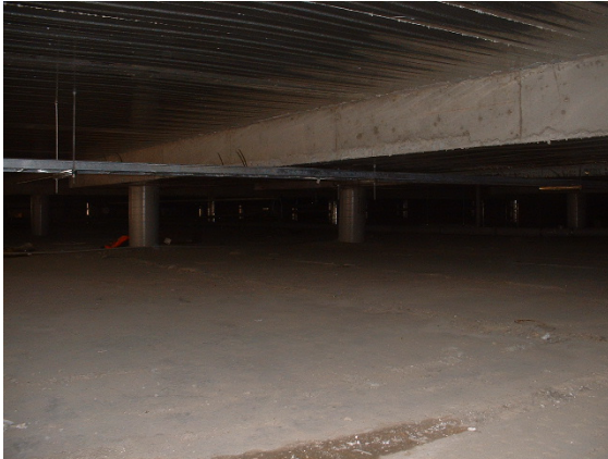
Figure 9 Large vented sub-slab void
