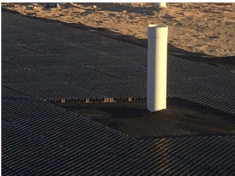
Figure 8 Modular drainage system installed beneath membrane
