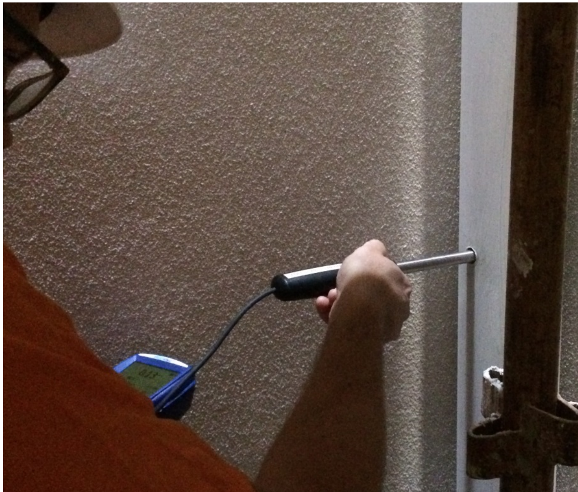
Figure 11 Measuring flow in a riser using hot-wire anemometer (TSI VelociCalc)
