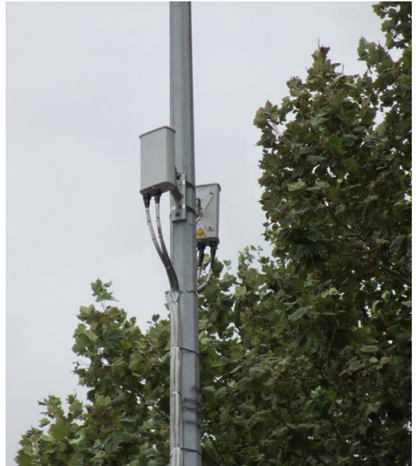
Figure 6 Microcells attached to a light pole.
