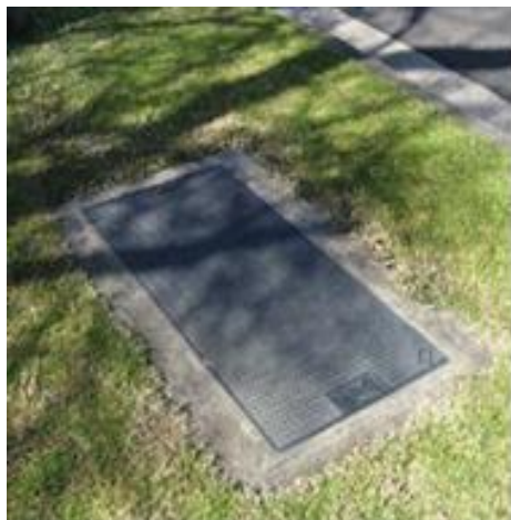
Figure 9 Underground housing for telecommunications facilities
