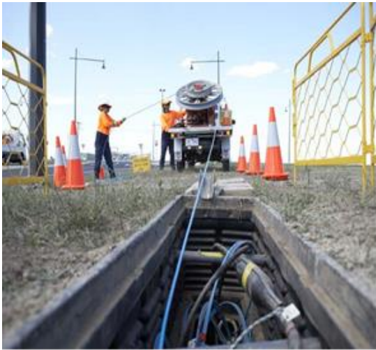
Figure 11 Cable being inserted into duct
